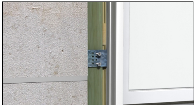
Figure 19 Attaching window with structural brackets.
